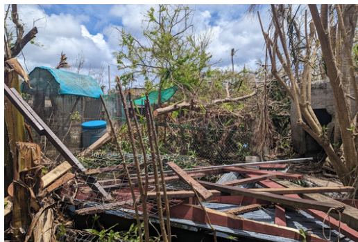
Guam Zoo storm damage
